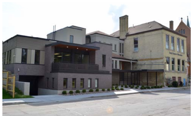
Last month the Guest House celebrated the completion of an 8,000 square foot addition (on the left in this photo). The new construction and renovations to the original building cost $2.8 million.
